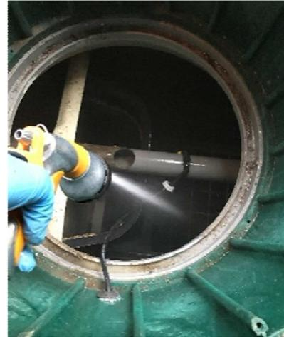
**Step 4. Insert suction hose into the baffle. Remove sludge from the bottom of Chamber 2. Rinse filtration media with pressure water during pumpout. This prevents the weight of loaded media in Chamber 2 from damaging the suspended platform on which it rests.**
