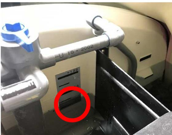
**Step 6. Refill water to the low water level (LWL) mark in all chambers immediately following all sludge pump-out operations. This operation is necessary to prevent tank damage or breaching from exterior pressure.**
