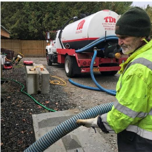
During pump-out, no vehicles of any kind (including the pump truck performing pump-out operations) shall be parked or located on the slab
