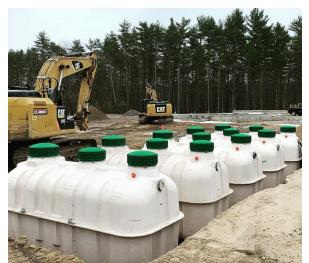
FujiClean systems may be cluster-configured to treat hydraulic flows of up to 100,000 gpd and organic loads of up to 3,000 mg/L BOD. Treated Effluent Aerobic Chambers Chamber Aerobic Contact Filtration Chamber
