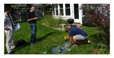
All onsite treatment systems must be maintained. But not all systems are created equal when it comes to maintenance. Fuji Clean systems are designed for exceptionally efficient servicing, which consists primarily of a routine flushback cleaning procedure managed by a technician simply turning valves. No filters are removed, no special equipment is required. Professional installers and maintenance providers tell us every day, "Easiest system to install and maintain ever!"
